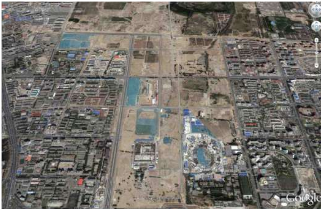
FIGURE 2: OLYMPIC GREEN, BEIJING . MAY, 2005. IMAGE FROM GOOGLE EARTH. This Image DEPICTS The site with most of the existing structures demolished.
