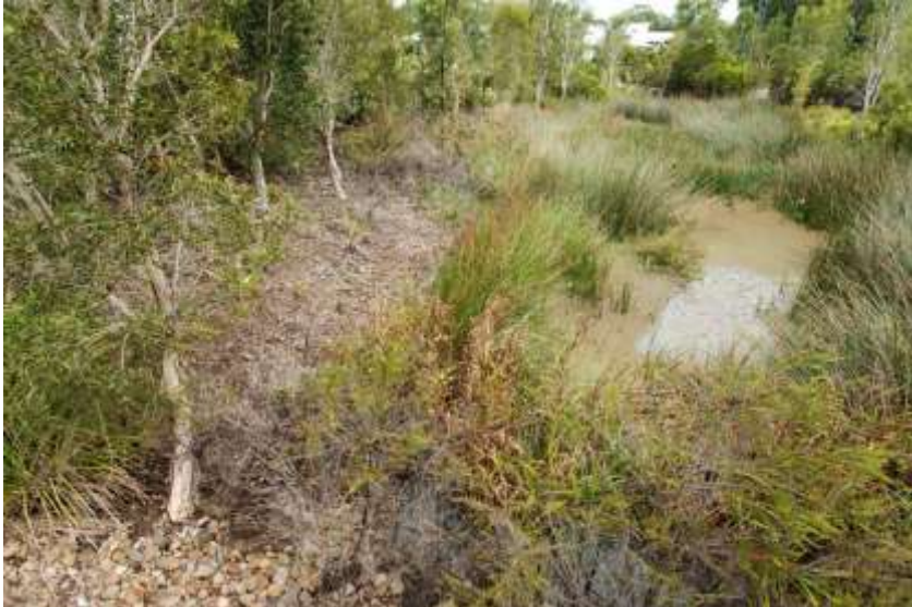
Figure 2 Stormwater treatment wetland
