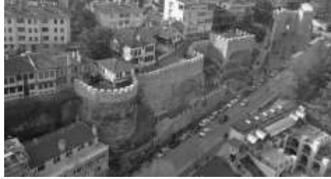
Figure 6. Restoration of city walls in the historic core
