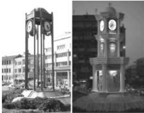
Figure 4. Heykel Clock Tower, before and after reconstruction
