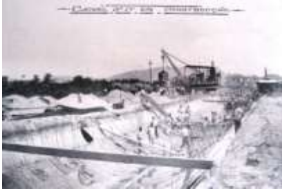
Figure 02 - Channel 4 under construction. Source: SÃO PAULO, 1925.
