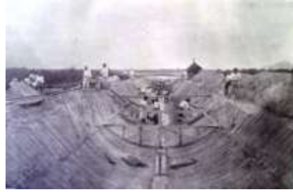
Figure 03 - Drainage channel 6 constructed with "Rodovalho cement". Source: SÃO PAULO, 1918.
