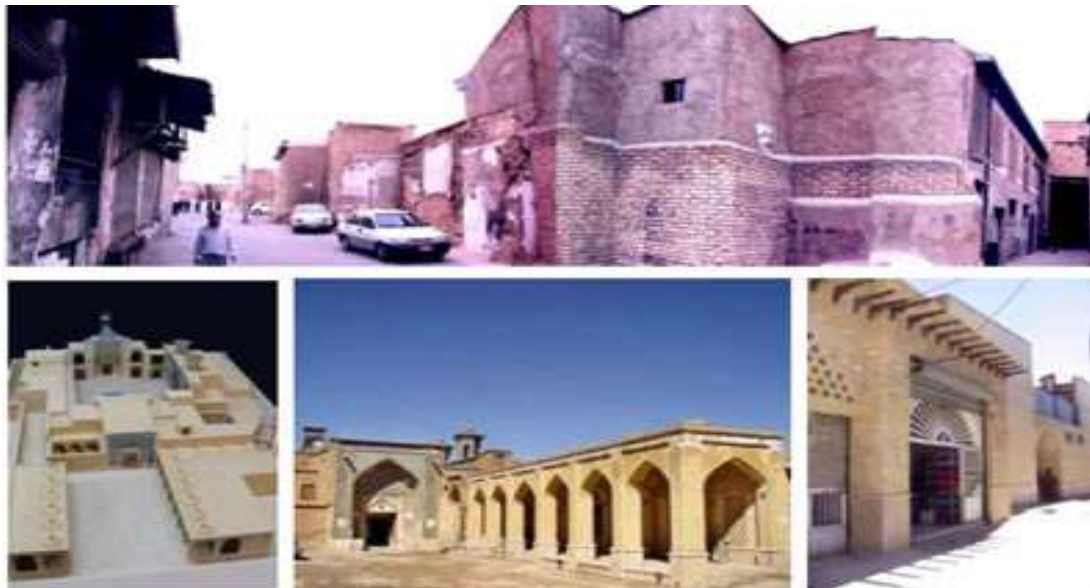
Figure 12 Moshir centre before and after regeneration. A group of low quality buildings were replaced by a new open space and shops located around the square. The new addition was constructed in a manner that preserved the historic character. While it was differentiated from the historic structure so that the new work is not confused with what is genuinely part of the past. The new element are compatible with the scale and future of the existing historic structures.
