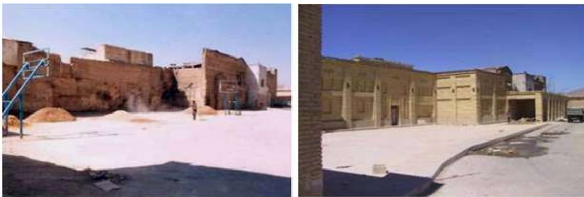
Figure 10 The view of sang-e siah axis before ( left ) and after ( right ) completion of the physical rehabilitation and open space improvement. In this project, the infrastructure improved, the main access resurfaced, and building facades were rehabilitated with the traditional patterns particularly those which located around the newly constructed plaza.
